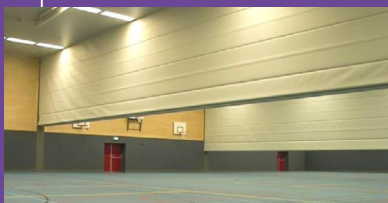
↑ Fireproof partition curtains with BasaTexx FP fabric in a sports hall
